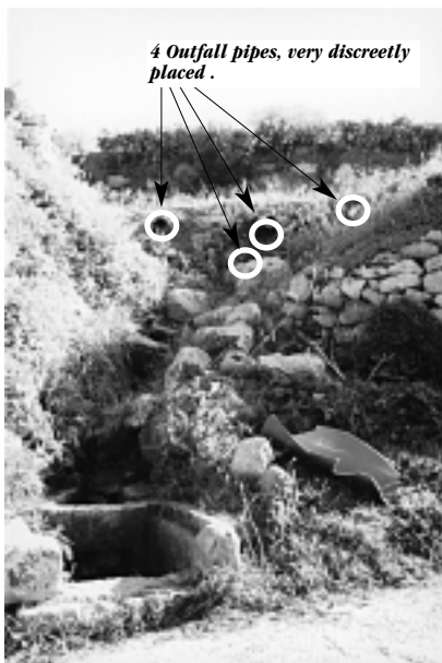
Fig. 3, Run-off pipes, situated just above Fig. 2 (2001): four pipes with outfall running down the rocks into the ‘watering’ hole at the bottom and on into the river system.
